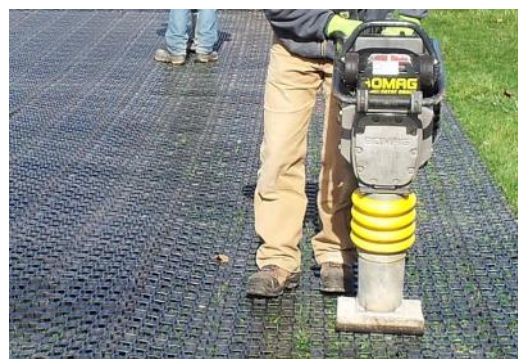
Rammer (trench compactor)
