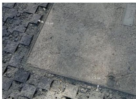
1-2 cm expansion gap should be left between the edge of the PERFO matting and immovable objects
