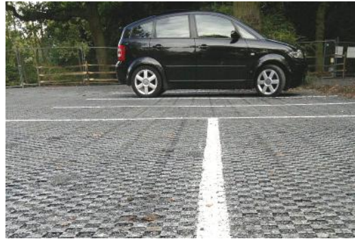
Line marking using highway marker paint
