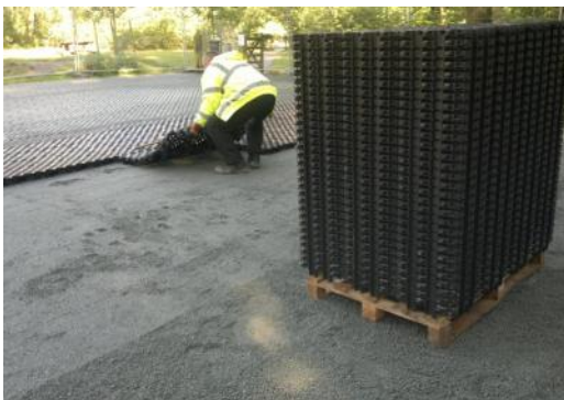
Laying out the PERFO-AK mats
