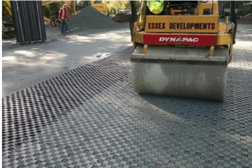
5 tonne tandem vibrating roller subsequently used for further compaction of the reinforced area.
