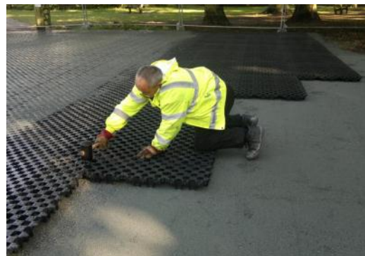
PERFO-AK mats being clipped together
