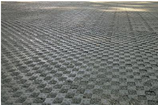
PERFO-AK after compacting into bedding layer
