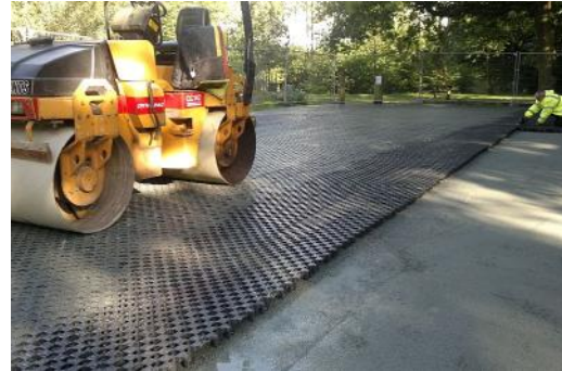
5 tonne tandem vibrating roller subsequently used for further compaction of the reinforced area.
